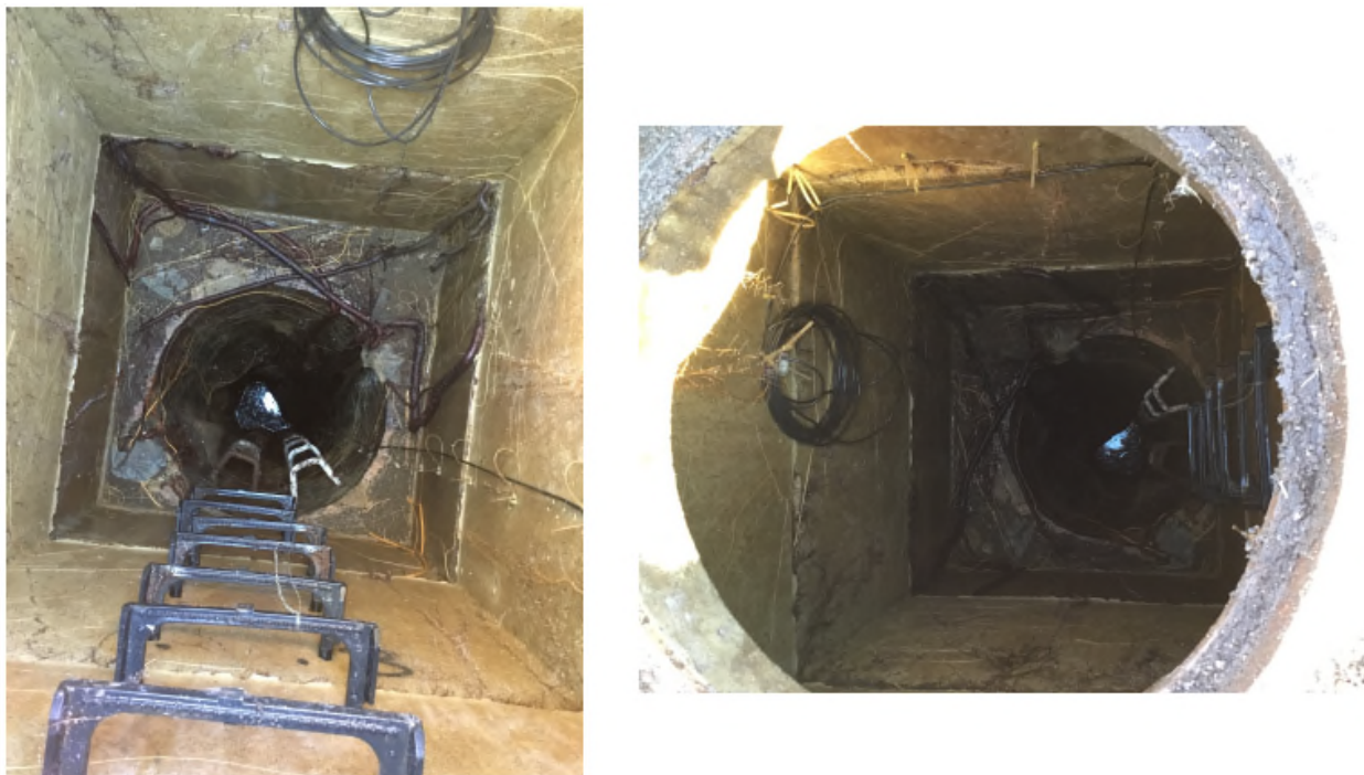
Figure 3-1: Downhole Photos of MH-4
